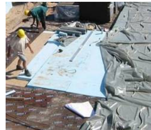
Fig. 3. 17 – Foamglas and XPS being installed under the floor slab of a five-storey office building
