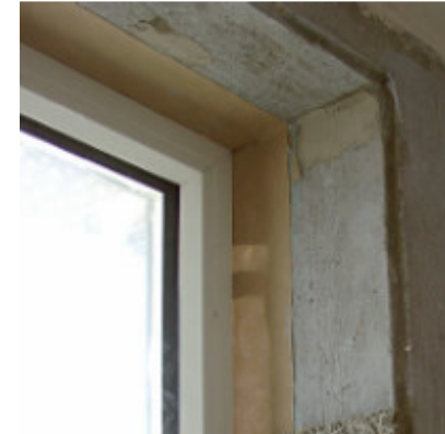
Fig. 3. 22 – The sealing tape, on which plaster can be applied, will then link the interior plaster and the window
