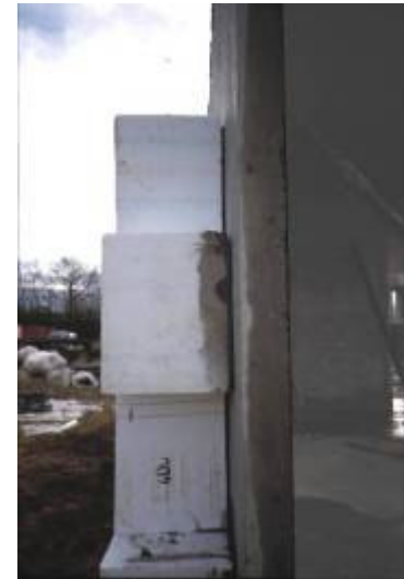
Fig. 3. 18 – 40 cm gable wall compound insulation system in a Passivhaus in Hannover
