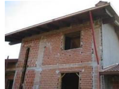
Fig. 3. 24 – Thermal bridges formed by concrete pillars and beams, in this case slightly reduced by two-hole hollow bricks
