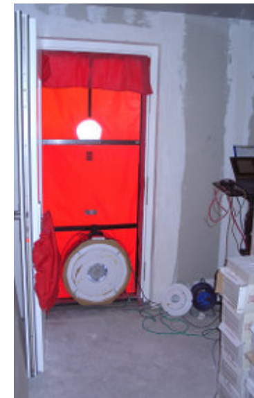
Fig. 3. 23 – Blower door installed for a pressurization test
