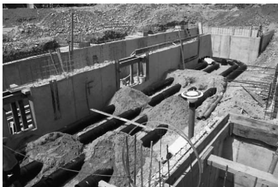
Fig. 2. Earth-to-air heat exchanger under construction, Fraunhofer ISE (Freiburg).
