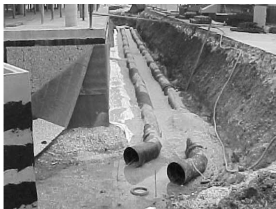
Fig. 3. Earth-to-air heat exchanger under construction, Lamparter (Weilheim).
